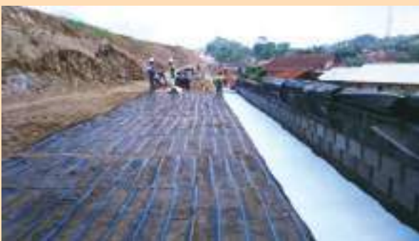
Pemasangan tensar multiblock STA 27+450 - 27+475 Tensar multiblock assembly SIA 27+450-27+475
