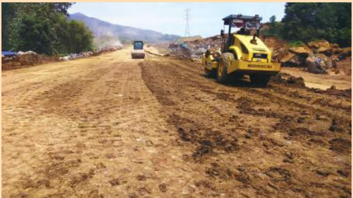
Pemadatan timbunan Ramp 3 Embankment compaction Ramp 3
