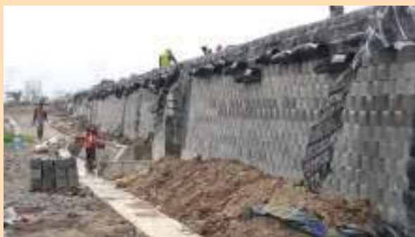
Retaining wall multi block STA 27 + 400
