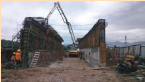
Pengecoran dinding BUP 1 Retaining BUP 1 wall
