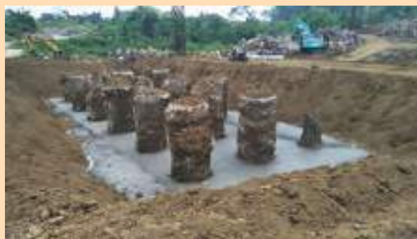
LC pile cap Abutment 1 OP IC cimilaka
