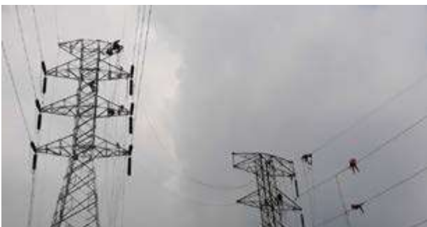
Proses pemindahan kabel konduktor dari tiang SUTT Eksisting ke tiang SUTT New dan sudah selesai pembongkaran tower Emergency The process of moving conductor cable from the existing SUTT to New SUTT and the completion of emergency tower dismantling.
