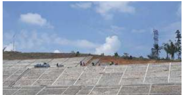
Dinding penahan lereng Slope retaining wall
