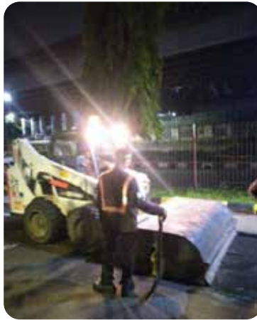
Lokasi perbaikan Scrapping Filling Aspal Rutin dilaksanakan spot by spot pada lokasi Off Ramp Kebon Nanas ruas North-South-Link . Asphalt patching maintenance were carried out spot by spot along the Off Ramp Kebon Nanas, North-South-Link section.
