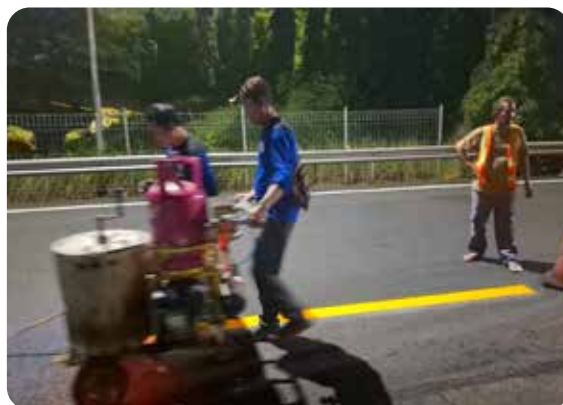
Lokasi perbaikan Marka Jalan Rutin di laksanakan spot by spot pada lokasi Interchange Cawang Arah Grogol-Posko Cawang ruas North-South-Link . The Routine Road Marking maintenance were carried out spot by spot at Cawang Interchange to Grogol-Cawang Post, North-South-Link section.
