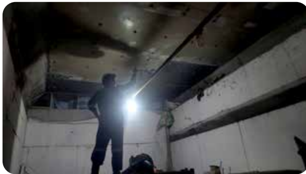
Lokasi pekerjaan Pengecatan perkuatan Steel Plate Bonding dilaksanakan pada lokasi segmen Gedong Panjang ruas Harbour Road . The painting of Reinforced Steel Plate Bonding was carried out at Gedong Panjang segment of the Harbor Road section.
