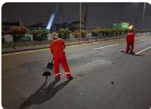
Lokasi perbaikan Patching Aspal di laksanakan spot by spot pada lokasi Ruas North-South-Link & Harbour Road Asphalt patching maintenance were carried out spot by spot along the North-South-Link & Harbor Road sections.
