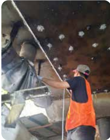
Lokasi perbaikan Injeksi Epoxy Perkuatan Steel Plate Bonding di laksanakan pada lokasi segmen Gedong Panjang ruas Harbour Road . Epoxy Injection of Reinforcement Steel Plate Bonding was carried out at Gedong Panjang segment of the Harbour Road section.
