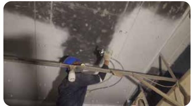
Lokasi pekerjaan Pengecatan perkuatan Steel Plate Bonding dilaksanakan pada lokasi segmen Gedong Panjang ruas Harbour Road . The painting of Reinforced Steel Plate Bonding was carried out at Gedong Panjang segment of the Harbor Road section.
