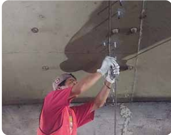
Lokasi perbaikan Injeksi Epoxy Perkuatan Steel Plate Bonding di laksanakan pada lokasi segmen Gedong Panjang ruas Harbour Road . Epoxy Injection of Reinforcement Steel Plate Bonding was carried out at Gedong Panjang segment of the Harbour Road section.
