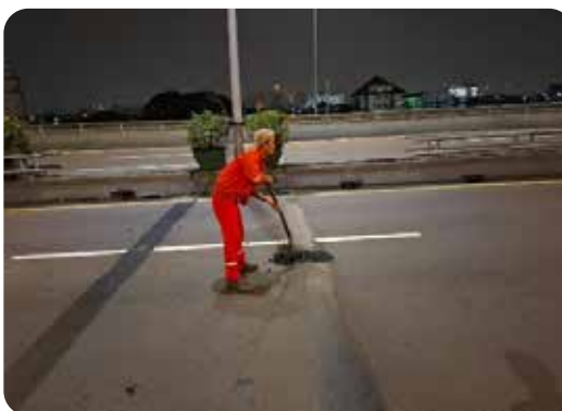
Lokasi perbaikan Patching Aspal di laksanakan spot by spot pada lokasi Ruas North-South-Link & Harbour Road Asphalt patching maintenance were carried out spot by spot along the North-South-Link & Harbor Road sections.
