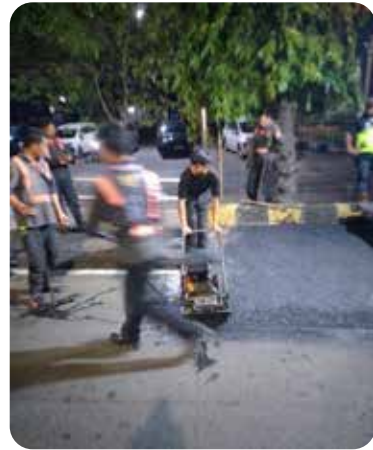
Lokasi perbaikan Scrapping Filling Aspal Rutin dilaksanakan spot by spot pada lokasi Off Ramp Kebon Nanas ruas North-South-Link . Asphalt patching maintenance were carried out spot by spot along the Off Ramp Kebon Nanas, North-South-Link section.
